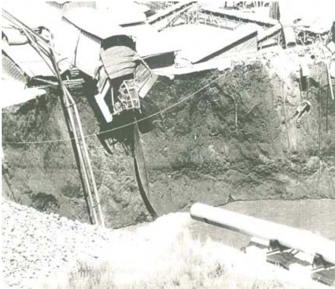
Visual 4: Sinkhole at the West Driefontein reduction plant in 1962
