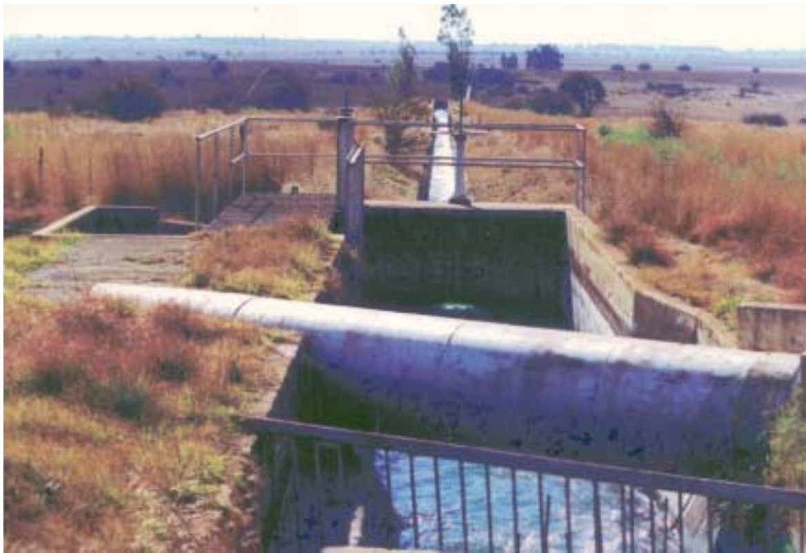
Visual 1: Water is piped across dewatered compartments to prevent pollution
