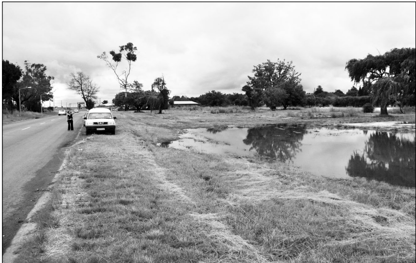
Figure 4: Small surface dam of raw sewage near the D field potable water abstraction boreholes and 300m from the municipal offices in Delmas
